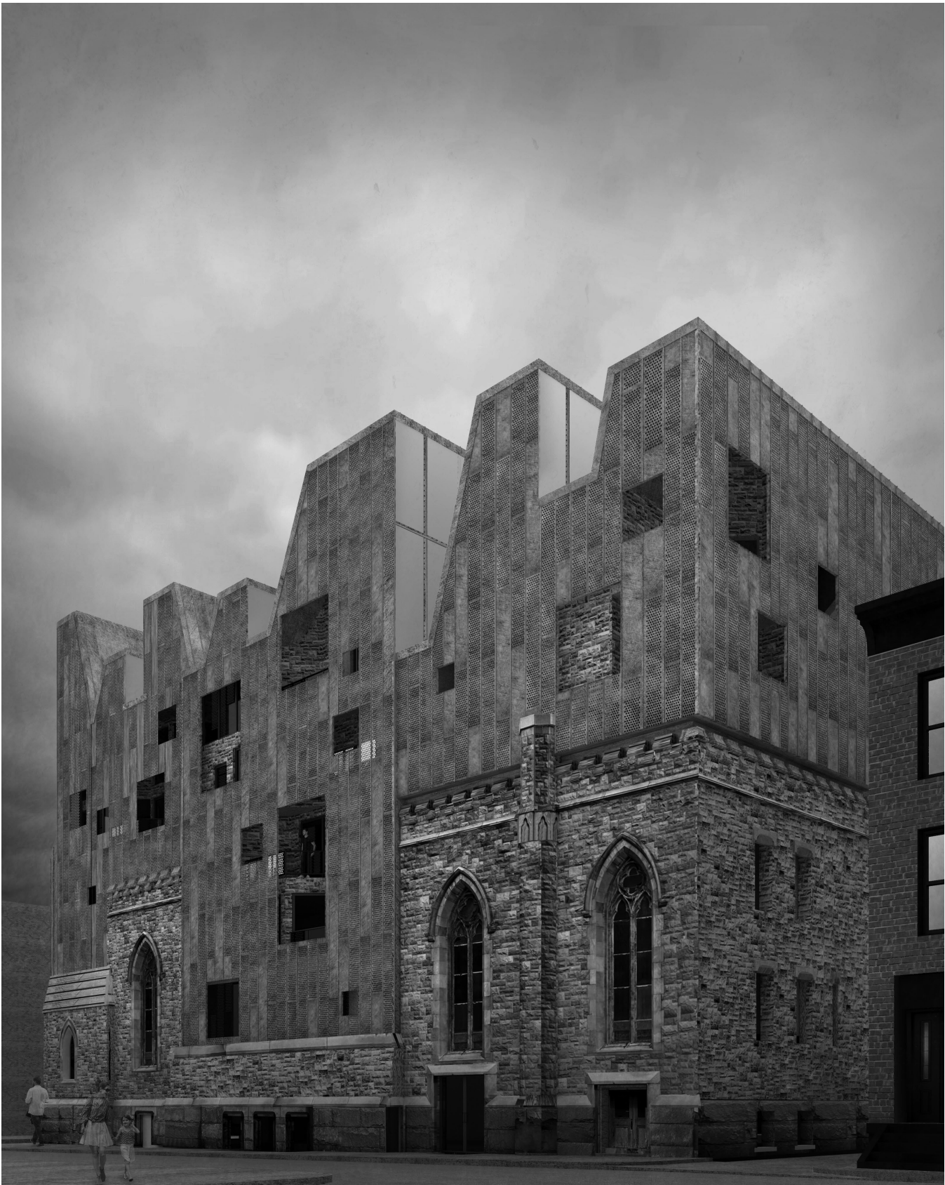
Figure 5. The housing addition atop St. Mary's church includes a perforated rainscreen and light monitors. The balconies and alcoves are finished with the repurposed stone facings from the church. Image by Erica Eom & Sarah Weber, RPI SOA, AD4, 2021.
